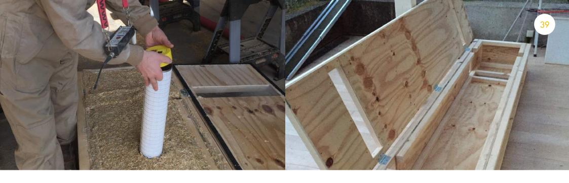
By that time ISO-Stroh had carried out their first cooperative tests with a German producer of blowing equipment, X-floc and they did a speed test on their straw, reaching more than 12 m³ per hour. By estimating about 10 m³ per hour as the maximum speed for local straw, we could estimate the time needed to fulfil the Tilburg project. When we added all the handling time at 50%, we could fill the straw, with 2 machines, at a rate of 10 m³ per hour.
